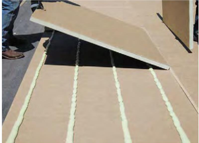
mopping and adhesive attachment methods. The product also performs well with mechanical fasteners.
