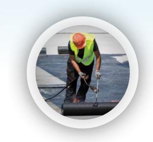
IKO Industries now offers the new ArmourBridge membrane system for bridge deck waterproofing layer applications. Made of a pre-formed SBS modified bitumen sheet, ArmourBridge is specifically designed for paving overburden and offers excellent protection for concrete structures against water-borne chemical deterioration.
