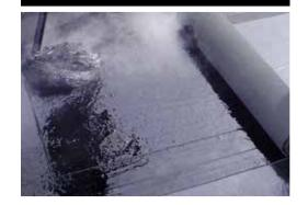
When used as a cap sheet, **Modiflex MP-180-SS-Base (3.0 mm)** satisfies the requirements of Type I, Grade S.
