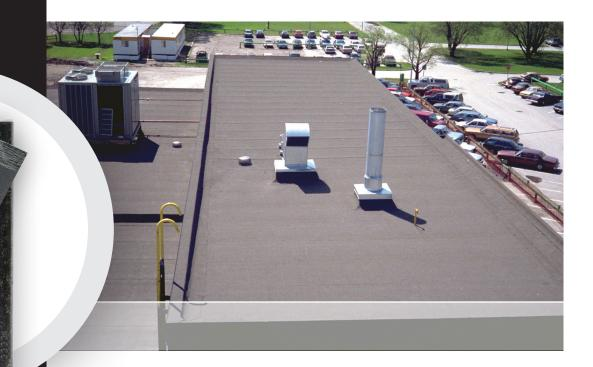
STOCK# 7361XXX ROLLS PER PALLET: 32 PALLET SIZE: 132 cm x 112 cm (52 in x 44 in) LENGTH: 8 m (26.24 ft) WIDTH: 1005 mm (39.6 in) AREA: 8 m<sup>2</sup> (86 ft<sup>2</sup>) THICKNESS: 4.2 mm (165 mils) SELVAGE: 90 mm (3.5 mils)
