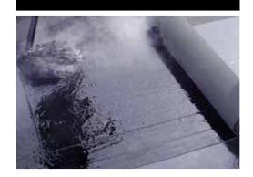
When used as a cap sheet, **Modiflex MP-180-SS-Base (3.0 mm)** satisfies the requirements of CGSB-37.56-M for Class P, Type 2 and Grade 2 materials as well as the requirements of ASTM D6164 for Type I, Grade S materials.
