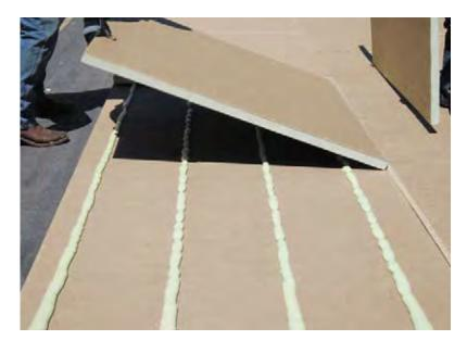
mopping and adhesive attachment methods. The product also performs well with mechanical fasteners.
