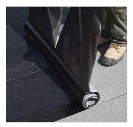
Tough ceramic colour coated granules protect the surface of the cap sheet.
