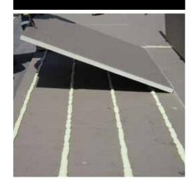
**IKOTherm Tapered** Commercial Roof Insulation satisfies the requirements of CAN/ULC S-704 for Type 2, Class 3 materials, and ASTM C1289 Type II, Class 1, Grade 2. This product is listed under CCMC listing #13037-L and is FM and UL approved.
