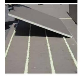
**IKOTherm Tapered** Commercial Roof Insulation satisfies the requirements of CAN/ULC 704.1 for Type 2, Class 3 materials, and ASTM C1289 Type II, Class 1, Grade 2. This product is listed under CCMC listing #13037-L and is FM and UL approved.
